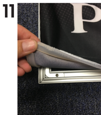
11 Make sure silicone is tucked beneath fabric.
