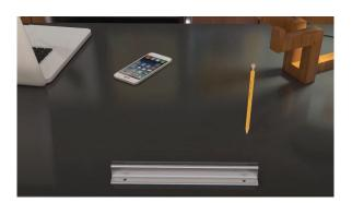
Place the channel in desired location and mark drill holes with a pencil; repeat for 2nd and 3rd channels (when applicable)
