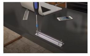
Line up channel holes with holes on surface and screw down. Screw for panel facing the inside
